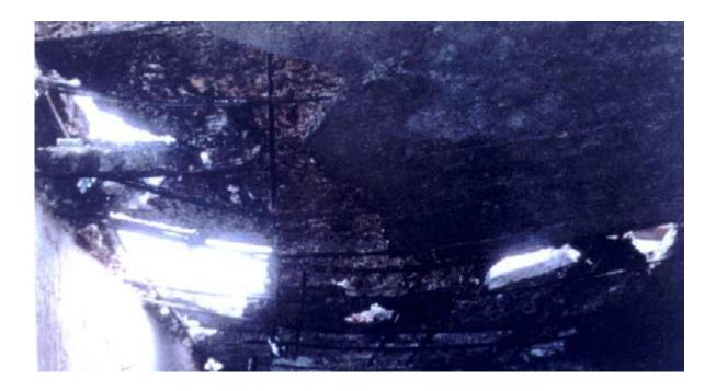
Figure 5: The above photograph depicts the ceiling region inside the bunker. Note the pieces of concrete missing, due in part to the spalling phenomenon. Also note that several large holes are present in the ceiling, not just a single circular hole in the center area of the roof.
