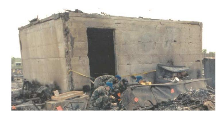
Figure 12: The above photo depicts the condition of the concrete bunker from the front side. Notice the cracks and pitting on the outside surface. There is enough space in front of the doorway to allow several men to work.
