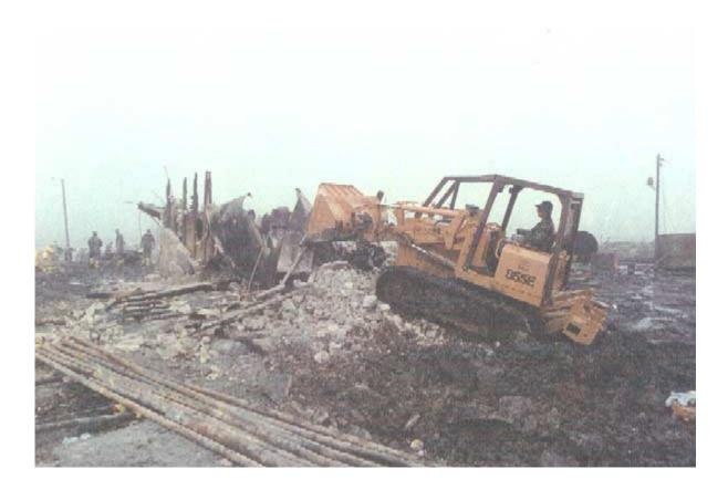
Figure 15: The photograph depicts the destruction of the concrete bunker. According to statements this was conducted due to the visibly and physically unsafe nature of the bunkers condition.
