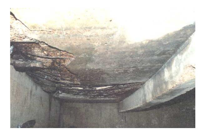
Figure 7: The above photograph depicts the extreme damage to the concrete on the ceiling of he bunker. Notice the "bowing of the ceiling and the pieces of concrete missing from the underside of the reinforcement bars.
