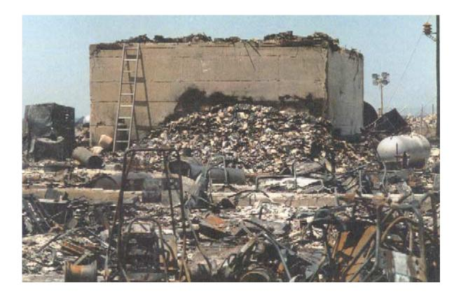
Figure 11: This photo depicts the back of the concrete bunker, note the condition of the concrete on the walls, with regard to cracks and pitting.
