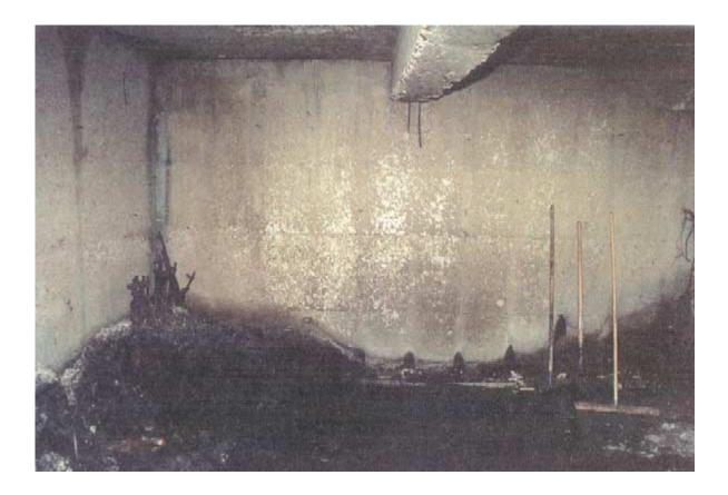
Figure 8: The above photograph again depicts the condition of the inside of the concrete, which constructed the bunker. Notice the pitting (missing pieces) on the concrete walls as well as the concrete beam in the ceiling.
