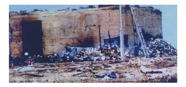
Figure 10: The above photograph depicts the front and side of the concrete bunker. Note the condition of the walls of the structure, specifically, the cracks and pitted areas located all over the outside walls.
