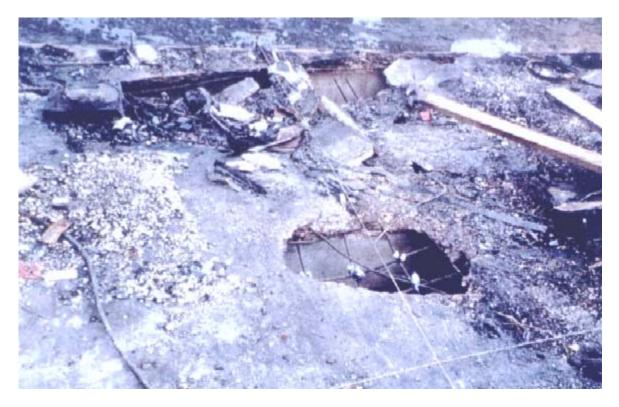
Figure 3: The above photograph depicts the circular hole located in the center of the bunker as well as several other hole located in the roof and their proximity to one another.
