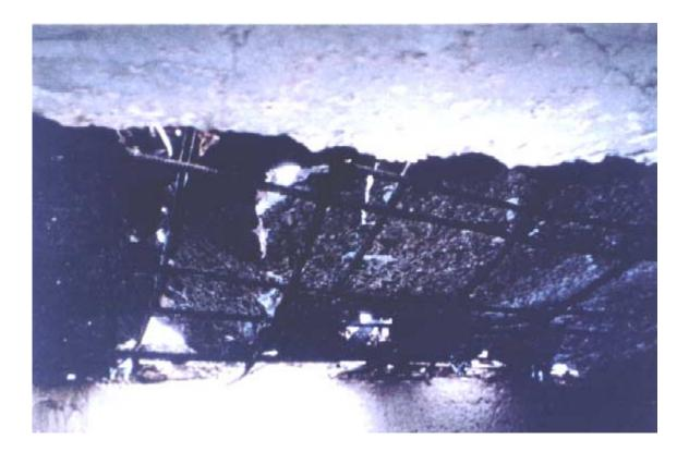
Figure 6: The above photograph depicts the ceiling region inside the bunker. Note the pieces of concrete missing, due in part to the spalling phenomenon. Also note that several holes are present in the ceiling, not just single circular hole in the center area of the roof.
