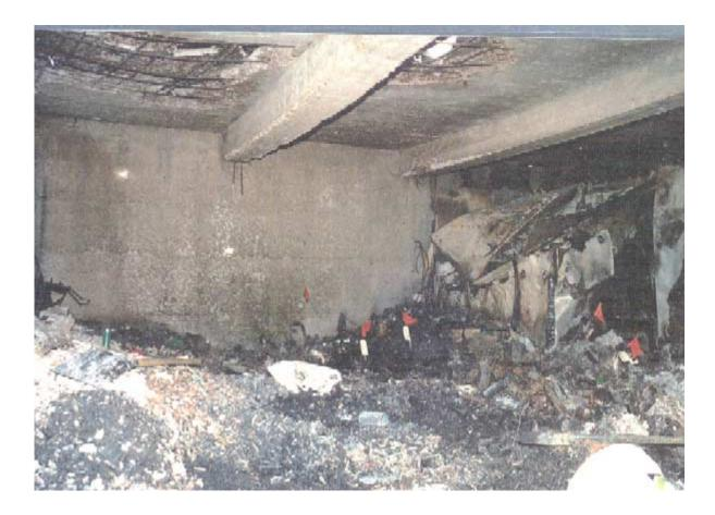
Figure 13: The photograph depicts the inside of the concrete bunker. Note the "bowing" of the concrete ceiling, the pitting or spalling of the concrete ceiling beams, the condition of the metal object along the wall. Notice the metal object, or cooler, is not directly under the hole in the center of the bunker roof.
