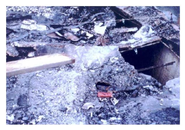
Figure 4: The above photograph depicts holes located in the roof of the concrete bunker. These holes occurred at the edge of the roof, several feet from the circular hole located in the center of the bunker roof (which can also be observed in figure 3).
