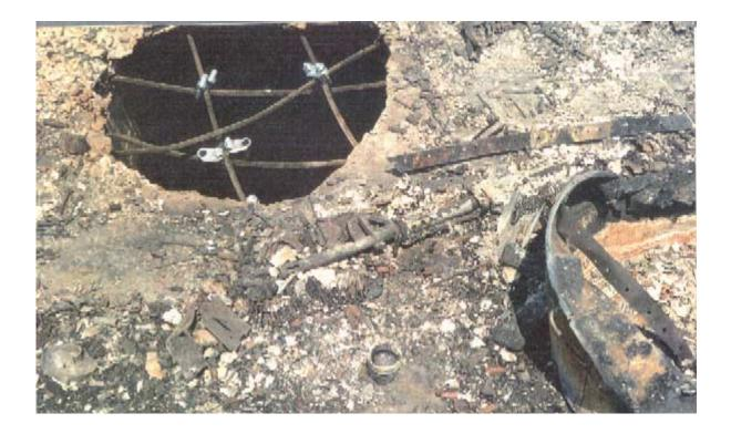
Figure 1: The above photograph depicts the questioned hole in the roof of the concrete bunker. Notice the four(4) u-bolts used on the reinforcement bars for safety precautions and the bowing of the reinforcement bars
